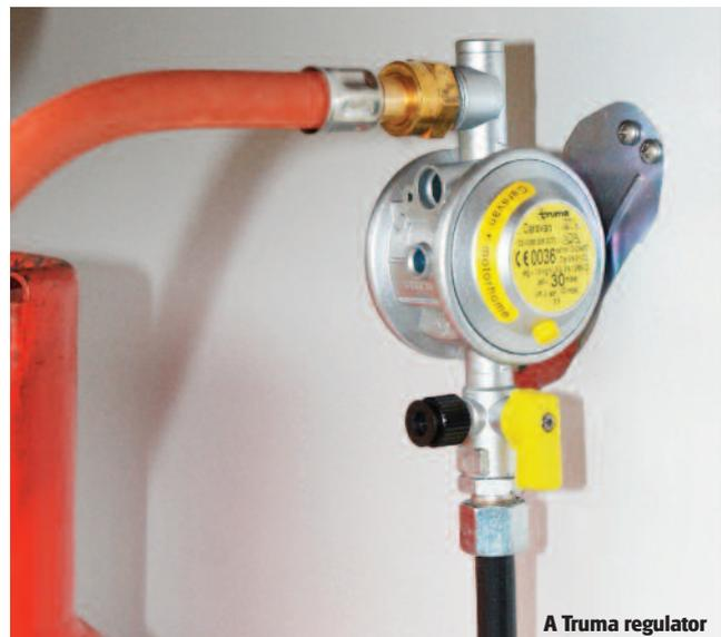
Perhaps more important though is to be sure the gas you have will supply all the appliances you want to have on at the same time. A single 6kg propane cylinder will have an available maximum off-take (supply) rate of up to about 0.8kg per hour. This will be sufficient for a cooker, space heater, fridge and water heater, but if you use all these and the grill and four gas rings at the same time you might find the cylinder cannot cope with the demand.
