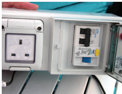
Use only proprietary hook up equipment with safety devices including a RCD and an IP rating of 44 or greater
