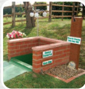
Suitable access must be available for cesspool and tank systems, to allow the sewage tanker to periodically empty the CDP collection vessel.
