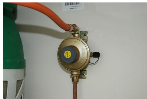
A bulkhead-mounted Clesse regulator
